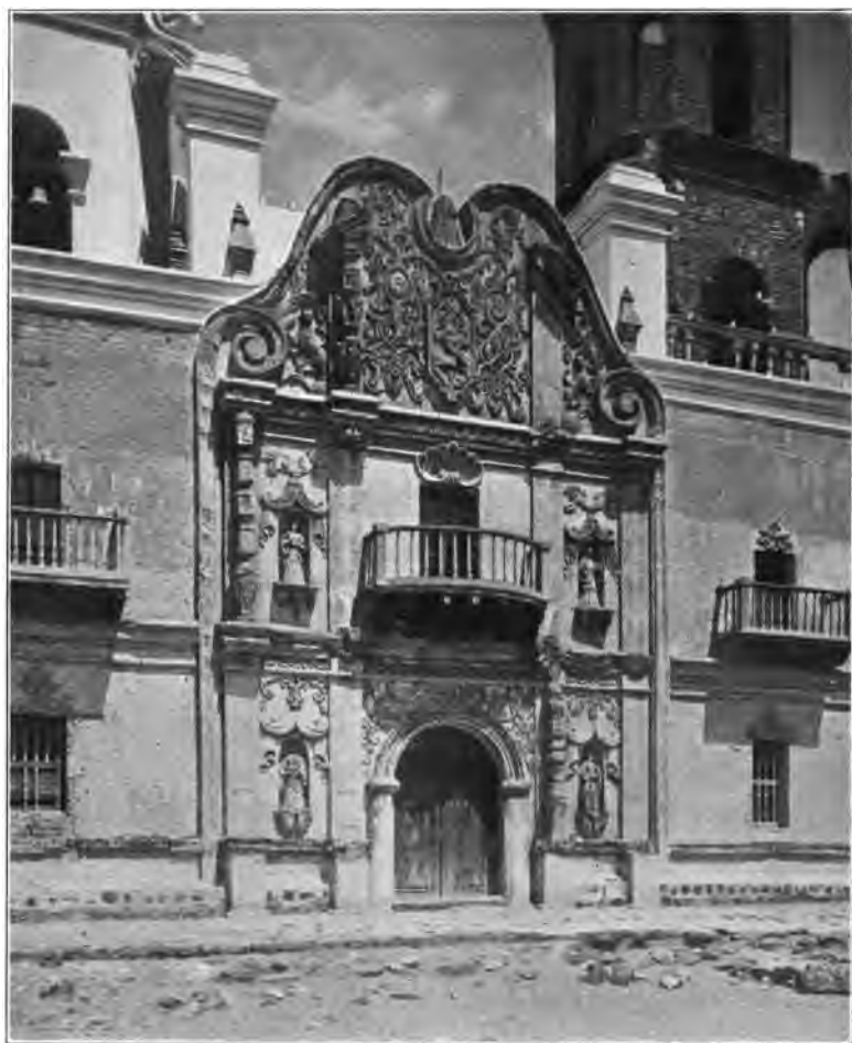
SAN XAVIER DEL BAC. Ornamental Gable about Main Entrance.
